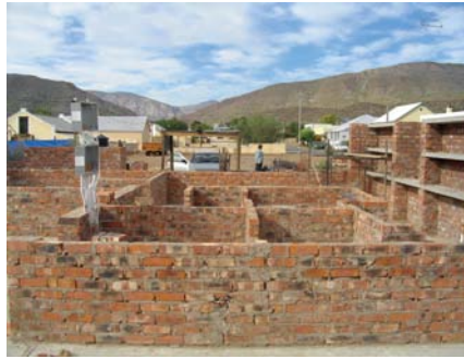
April 2012 The foundations are laid, the wall is at half-height and the built-in bookshelves are clearly visible on the right.
