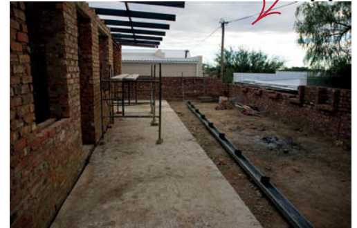
May 2012 The steel roof goes up and the concrete stoep floor in the courtyard is laid.
